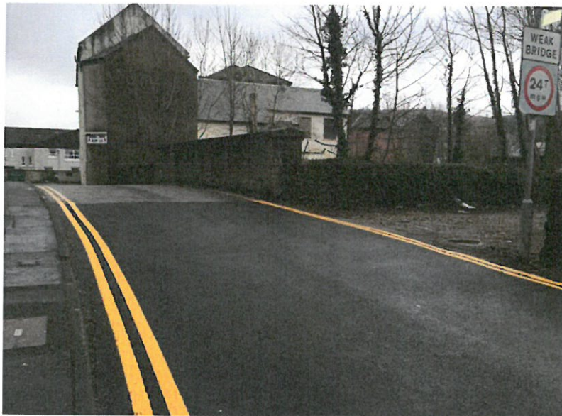
View of Site Entrance looking North East
